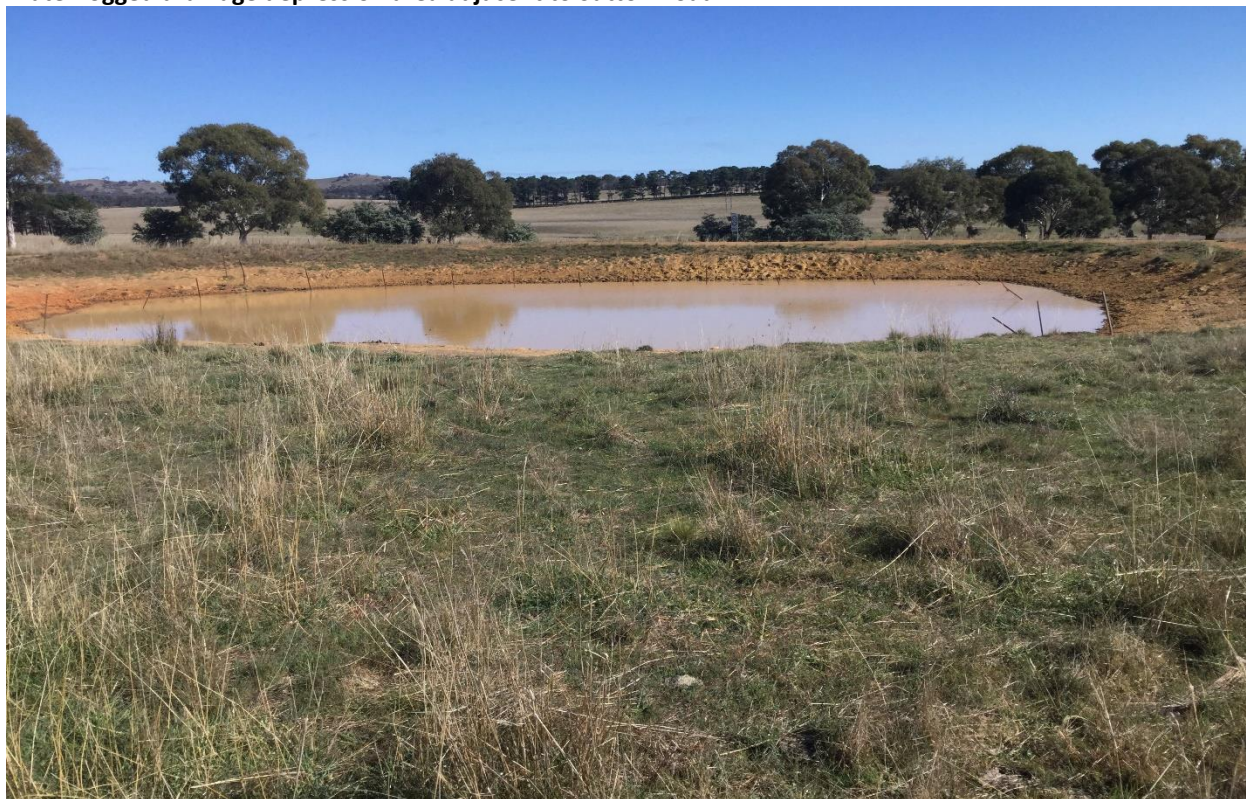
Erosion control dam in Extended Village Core area upslope of Sutton Road
